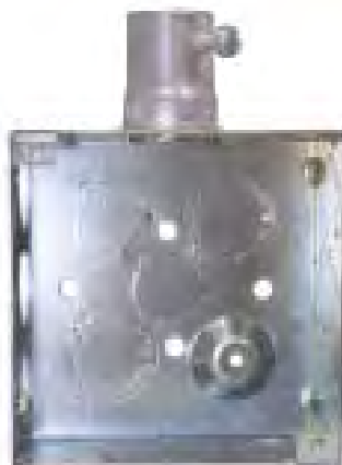
Twistlock box with a TL connector
